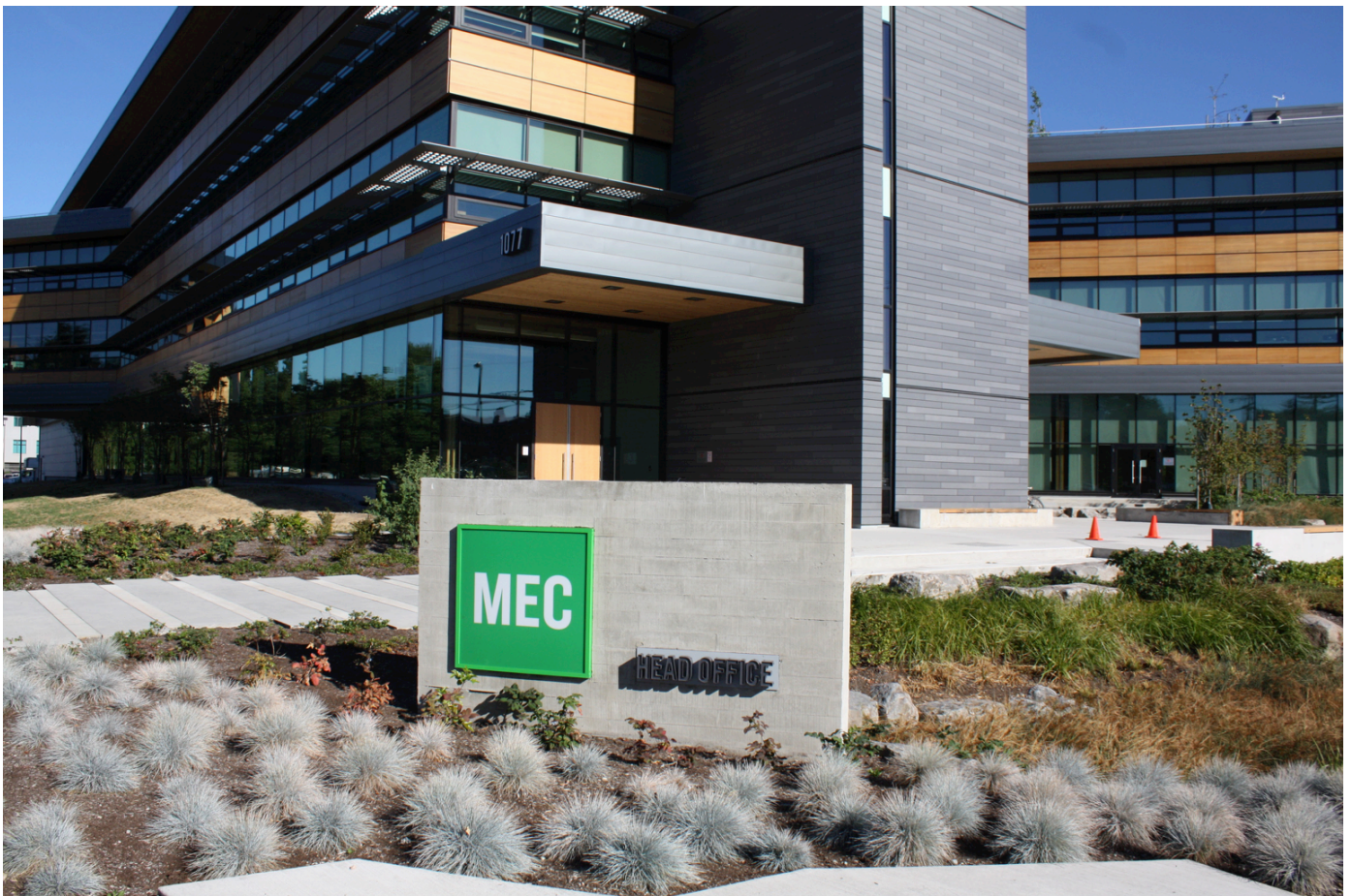
FLA staff conducted the MEC headquarter assessment in Vancouver, Canada in July 2015.
